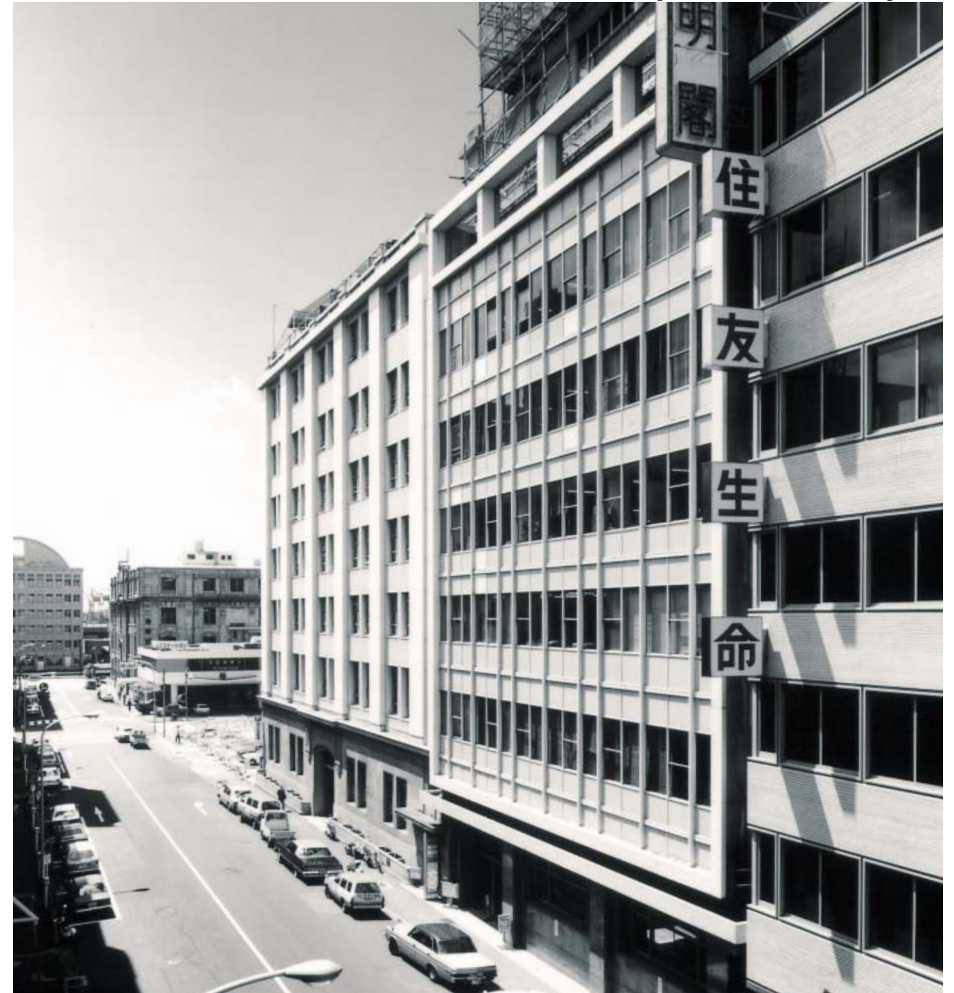
明海ビル新館増築後(1957年頃)／After building the new annex of the Meikai Building(1957)
